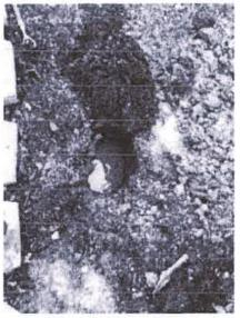
Performed sonic listening tests, leak noise heard in area where water is surfacing. Induced inert gas at hose bib in garage driveway. Conducted additional sonic listening in area leak noise was heard, water and gas was seen surfacing. Excavated to confirm location. Discussed results with customer onsite.
